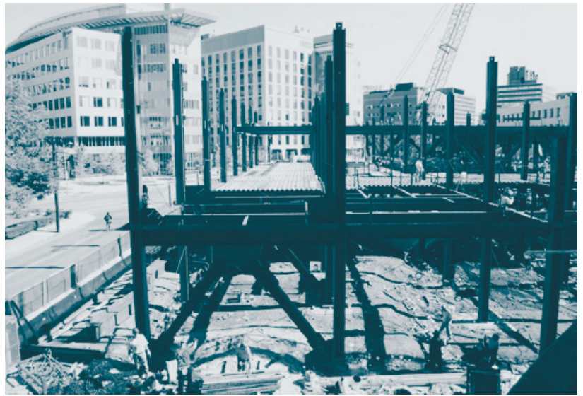
progress as of September 26
